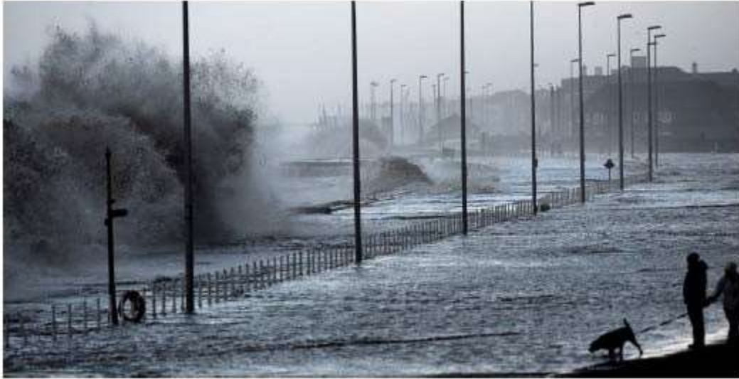
Figure 4.4 Wave overtopping at a seawall with a wide boulevard
