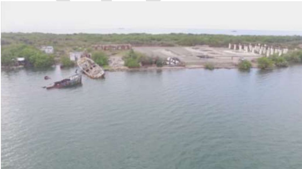
Figure 6.2-4. Shoreline conditions along the middle section.
