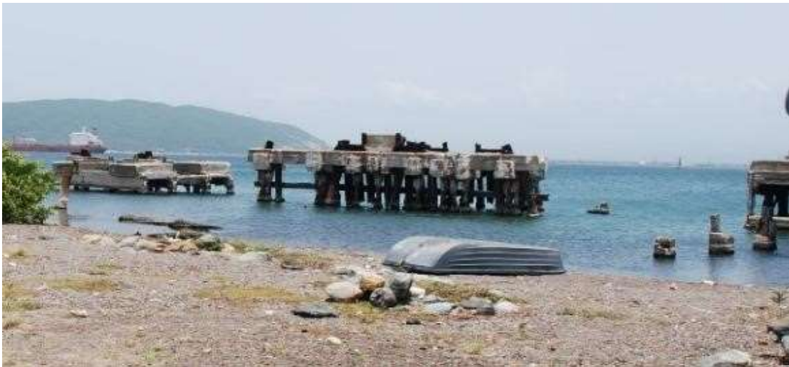
Plate 1. Remnants of modern concrete wharf element on the Old Coal Wharf property, 2015.
