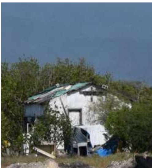
Plate 15 . A small degenerated concrete building
