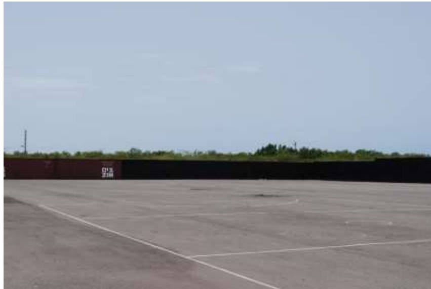
Plate 6. Showing a section of the asphalted surface at the Old Coal Wharf, JNHT photograph, 2009
