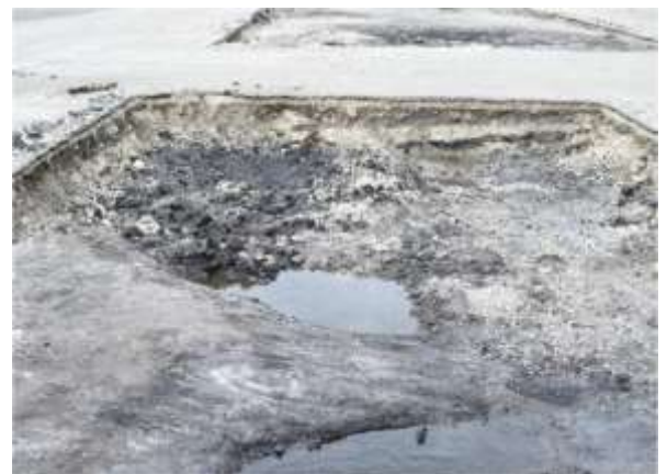
Plate 26. Test Trench 5 depicts brick commingled with concrete rubble and mangled iron bars.
